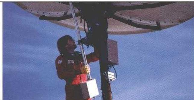
*Above, Curtis Mathes home satellite television installer prepares to mount actuator arm as he steadies antenna dish. Actuator assembly automatically positions dish to correct satellite.*
