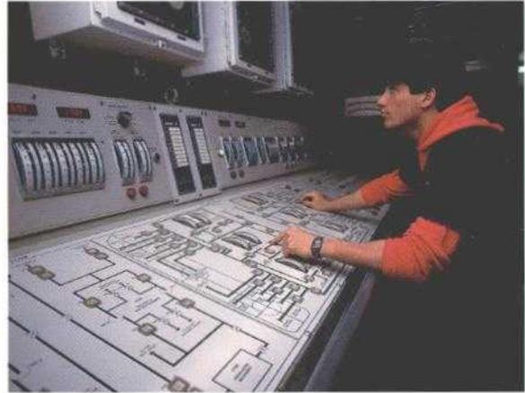
**Above,** In the ballast control room, crewman on duty constantly monitors the rig's stability and makes adjustments if necessary. **Below,** The John Shaw as seen from a supply ship. At least one such ship is always on station with a drilling rig.
