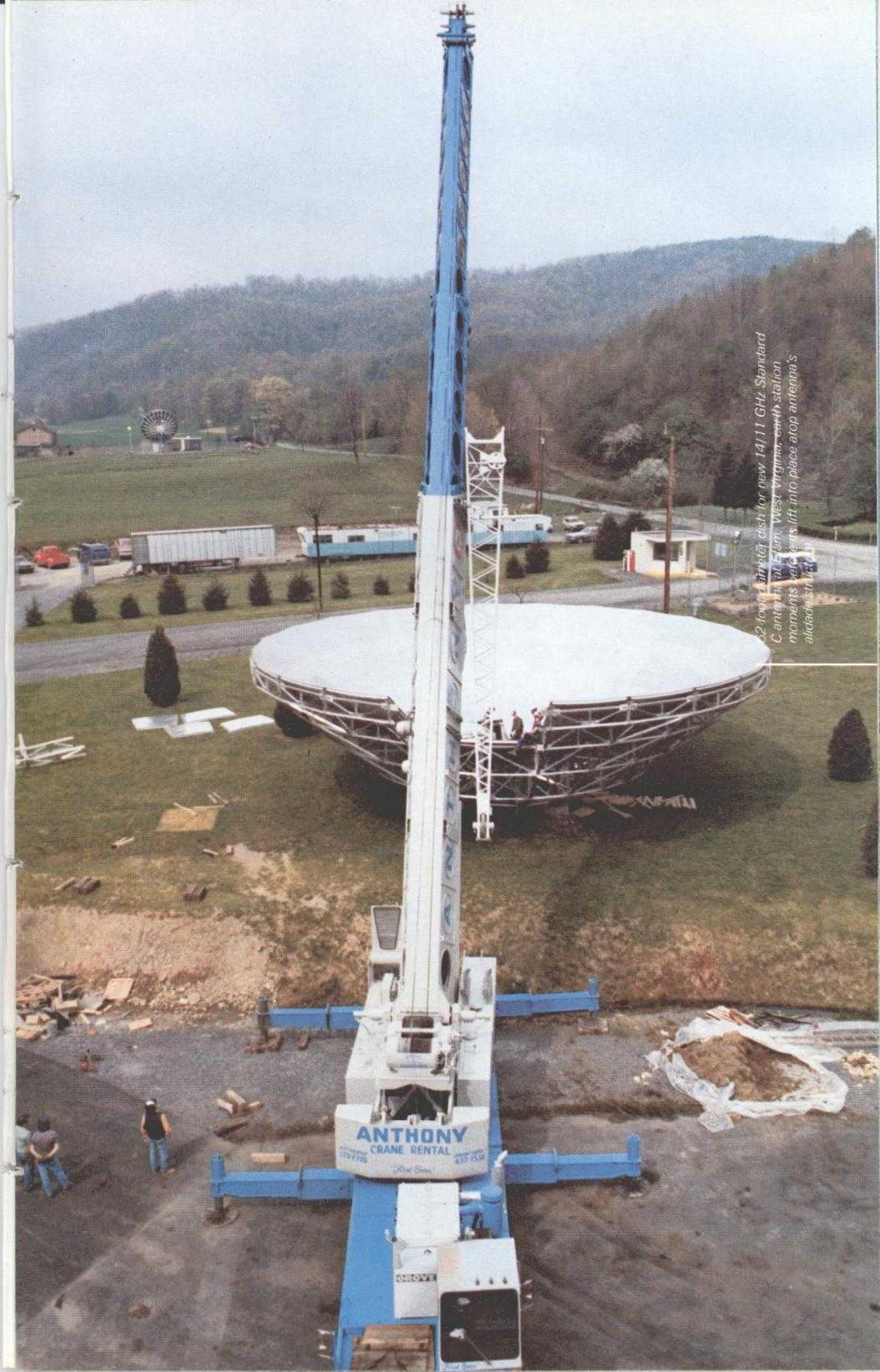
62-foot diameter dish for new 141.1 GHz Standard
